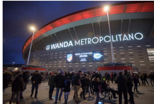
Picture 5: The spectacularly sweeping roof with integrated LED bands, the bright, horizontally perforated façade and the large-sized MEDIAMESH® display all blend in together perfectly.
