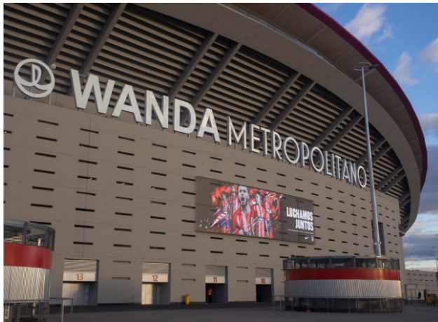
Picture 1: Six transparent Mediamesh®-panels from GKD, each measuring six meters high and four meters wide make up the visually seamless screen.
