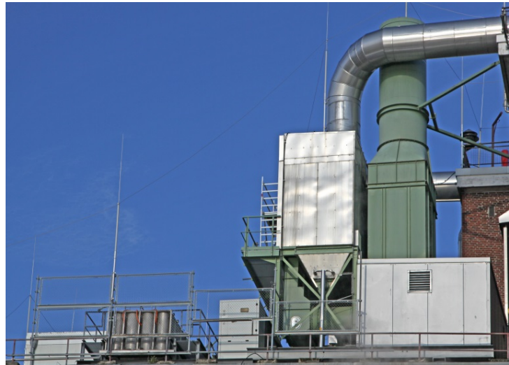
Picture 2: In hot gas filtration, the recovery of thermal energy after the filtration process not only dispenses with energy-intensive reheating of the exhaust gas, but also contributes to protecting downstream units.
