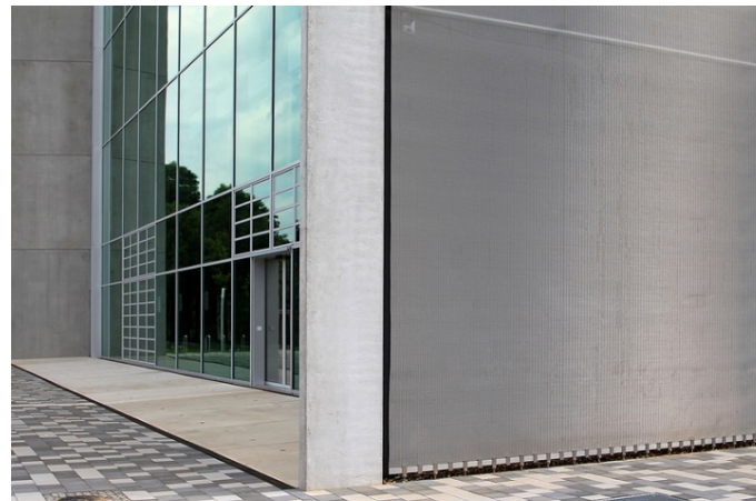
Picture 5: The lateral façades are spanned by a shimmering skin made of metallic mesh that creates a visually seamless surface.
