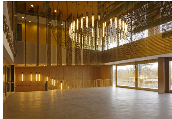
Picture 8: Perrault also relied on suspended objects and large-format wall hangings made of GKD metal fabric of the type ESCALE 7x1 for the design of the Salon Présidentiel .
