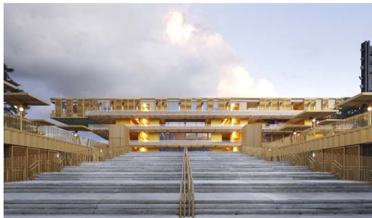
Picture 3: For the solar protection elements of the stand and pavilions that flank the main entrance golden stainless steel fabric of the type ESCALE 7x1.5 was used.
