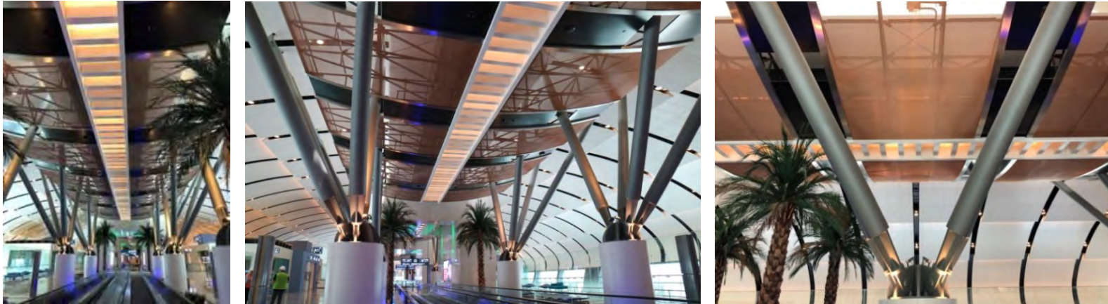
Picture 4-6: 210 fabric elements shimmering in a soft gold tone form semitransparent modern baldachins above the moving walkways flanked by large palm trees.
