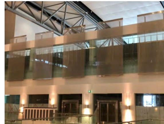
Picture 8-9: In the retail area in the third wing, stainless steel fabric from GKD provides decorative highlights in the form of large-scale wall-hangings.
