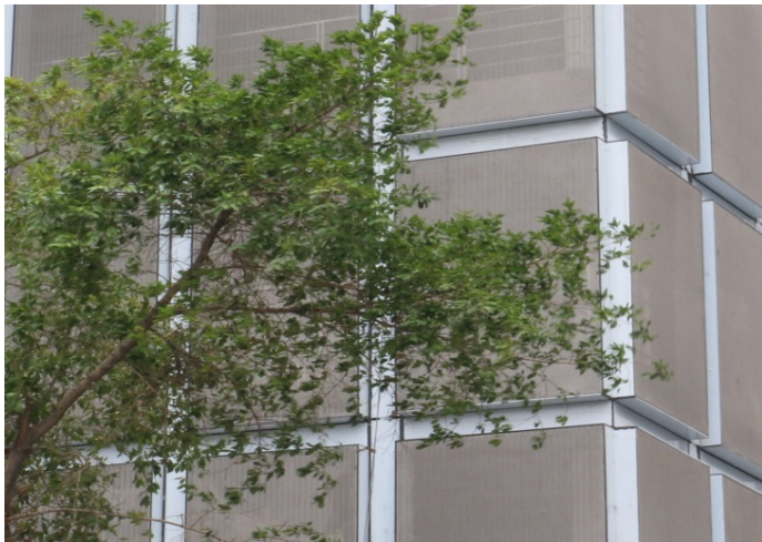
Picture 2: In order to adapt the parking tower's appearance to the luxurious overall ambience, the shimmering PC-Sambesi made of stainless steel mesh from GKD was chosen for the cladding.
