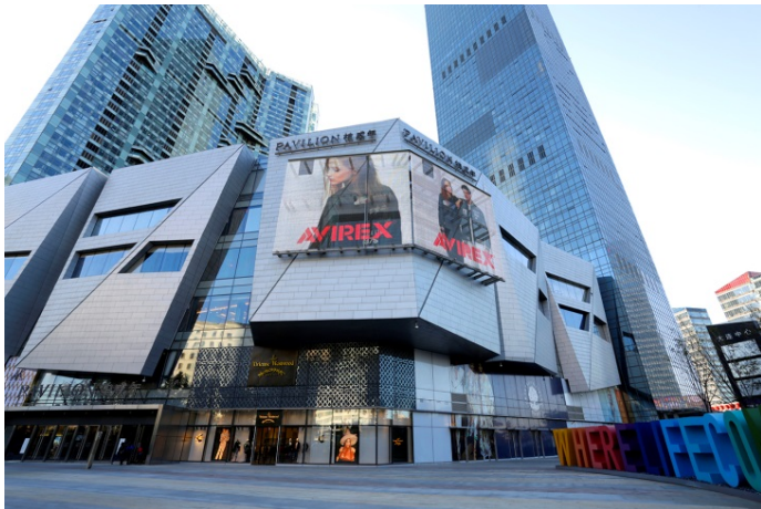
Picture 1: Large transparent MEDIAMESH® screens from GKD running around the corners of the building seize the attention of passers-by at both main entrances of Eton Place Dalian.
