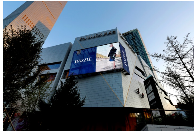
Picture 2: The transparent displays made of filigree stainless steel mesh with integrated LED profiles function as an advertising platform for luxury goods from all over the world and underline the exclusivity of the building complex.
