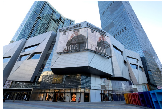
Picture 4: The transparency of the woven textile ensures that daylight can reach the rooms behind the media façade.
