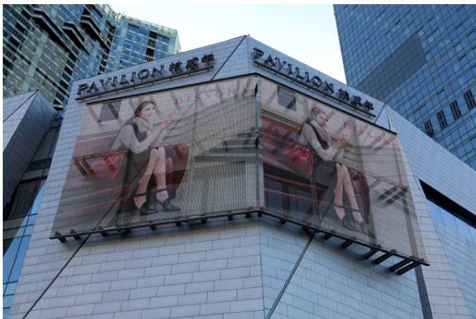
Picture 3: The two screens from GKD are 10.35 meters high and up to 24 meters wide, running over the corner at two entrances and – depending on what is being presented – allowing media to be viewed over an angle of 90°.
