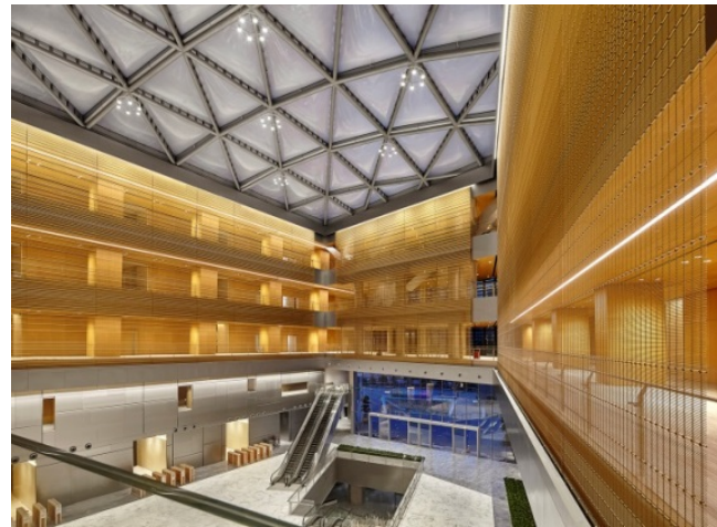
Picture 11: A total of 1,850 square meters of metal fabric from GKD is used to create a golden net that encapsulates the three-floor atrium of the Headquarter of the Chinese internet giant Tencent.
