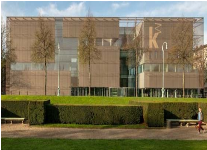
Picture 10: A shell made of bronze-colored stainless steel fabric from GKD lends the Kunsthalle Mannheim a distinctive face.
