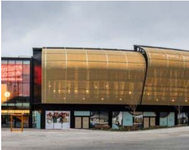
Picture 9: The way in which their properties combine predestines them for façade or ceiling projects, here as a façade cladding of the type PC-Alu 6010 of Elwick Place in London.
